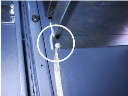
*Figure 6. Grounding strap secured to dispenser tray mounting bolt.*
