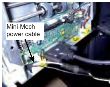
The DC power cable connection at the Mini-Mech dispenser.
