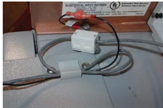
Figure 19. Secure excess cable.
