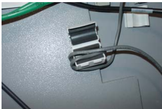
Figure 17. Install cable in ferrite.
