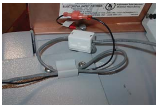
Figure 19. Secure excess cable.
