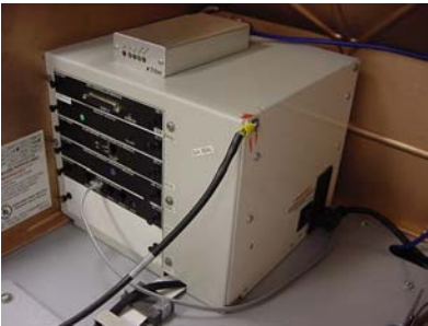
Figure 2-17. RS-232 cable routed.
