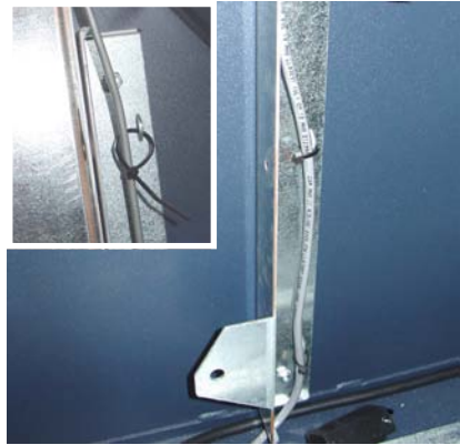
Figure 7. Route power cable behind bracket and secure with ty wraps.
