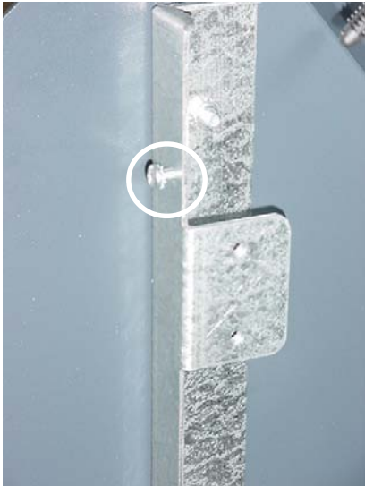
Figure 3. Screws started, not tightened.
