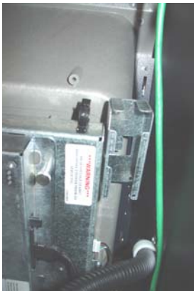
Figure 1. Remove screw/bracket.
