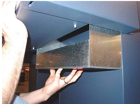
Figure 7. Remove plate.
