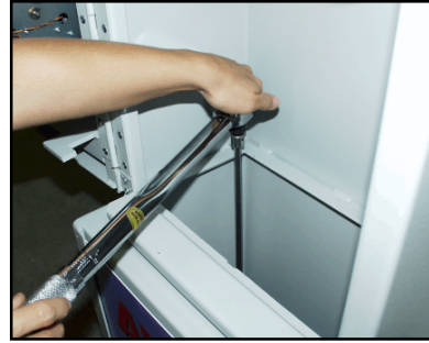
Fig. 9. Tightening Anchor Bolts (Preferred Method).
