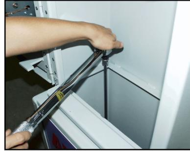
*Fig. 9. Tightening Anchor Bolts (Preferred Method).*
