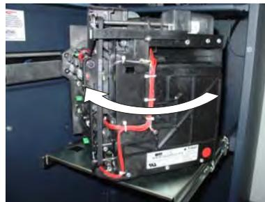
Figure 7. Rotate mechanism "clockwise".
