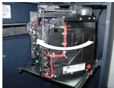
Figure 7. Rotate mechanism "clockwise".
