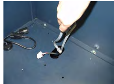
Figure 5. Feed cables down to vault area.
