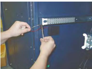
Figure 10. Remove door ground bolt.
