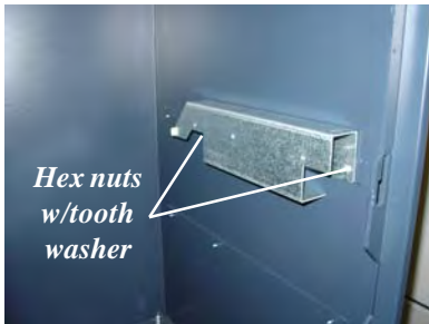
Figure 11. Side rails removed.
