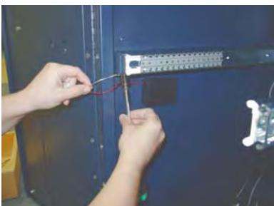
Figure 10. Remove door ground bolt.
