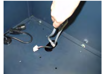
Figure 5. Feed cables down to vault area.
