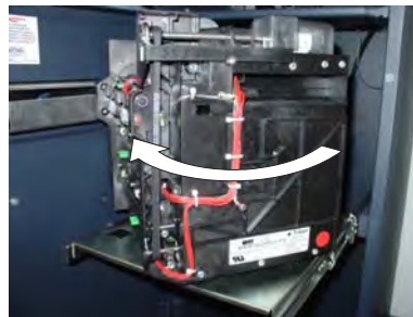
Figure 7. Rotate mechanism "clockwise".
