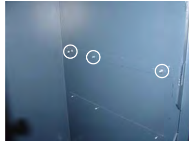
Figure 12. Nuts started on bolts.
