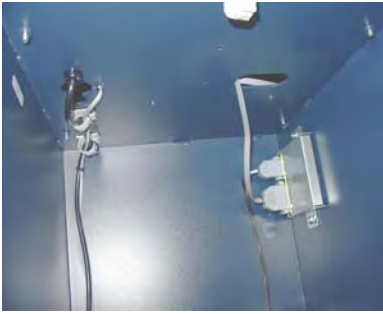
Figure 12. EJ to Docking board cable.
