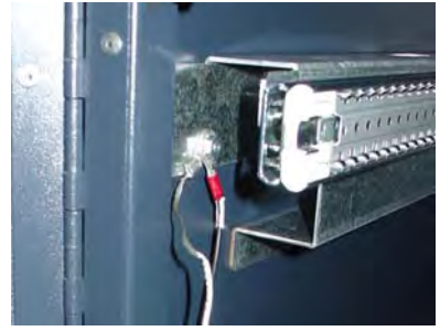
Figure 9. Ground wires installed.
