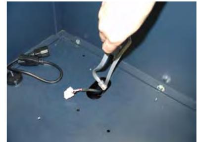
Figure 5. Feed cables down to vault area.
