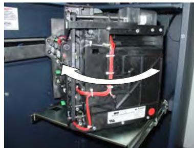
Figure 7. Rotate mechanism "clockwise".
