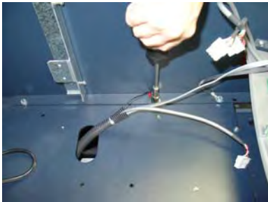
Figure 3. Disconnect ground wire.
