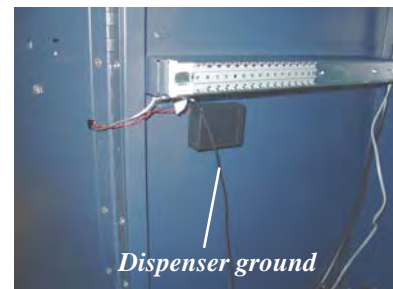
Figure 11. Dispenser ground installed.
