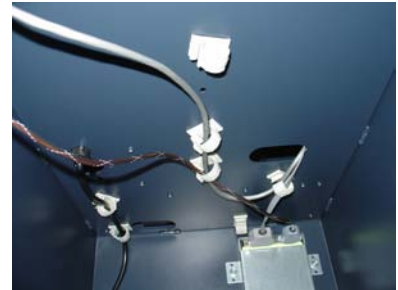
Figure 11. Route power/data cables.
