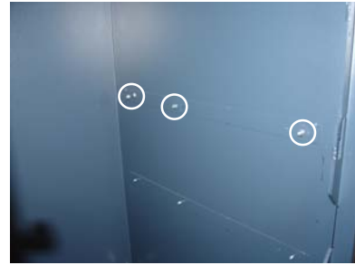
Figure 12. Nuts started on bolts.
