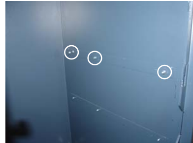
Figure 12. Nuts started on bolts.
