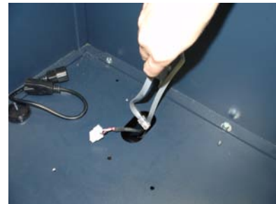
Figure 5. Feed cables down to vault area.
