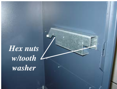
Figure 11. Side rails removed.
