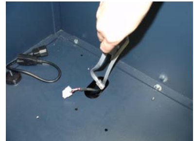
Figure 5. Feed cables down to vault area.
