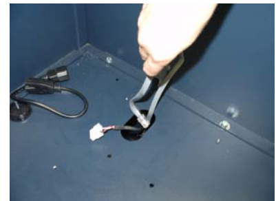
Figure 5. Feed cables down to vault area.
