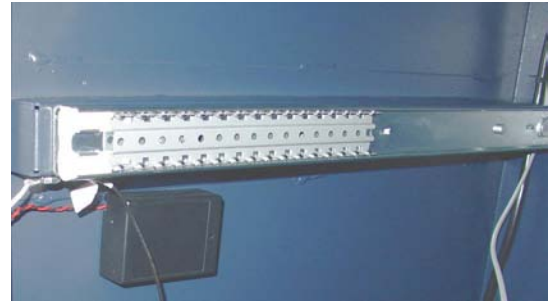
Figure 6. Slide rail installed.
