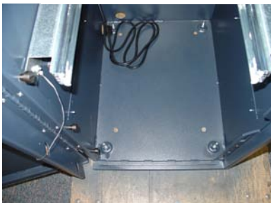
Figures 7 and 8. Slide rails flush w/bracket front.
