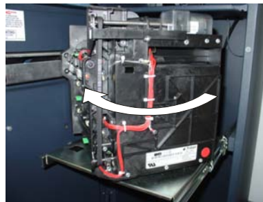
Figure 7. Rotate mechanism "clockwise".
