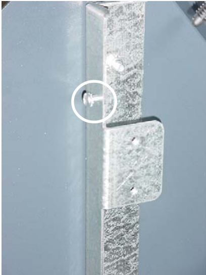
Figure 3. Screws started, not tightened.
