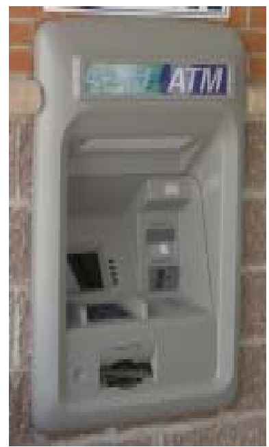
Slide unit back flush to wall.
