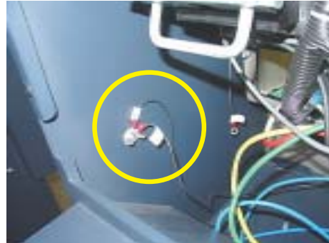
Secure ground wire.
