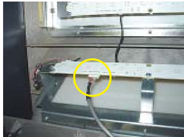
Secure ground wire.
