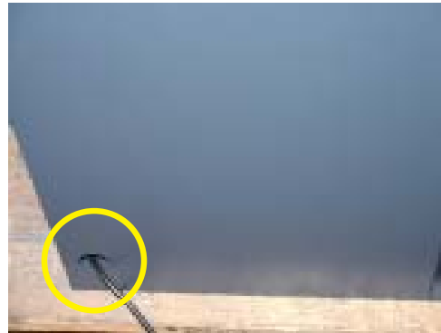
Left front side access hole.
